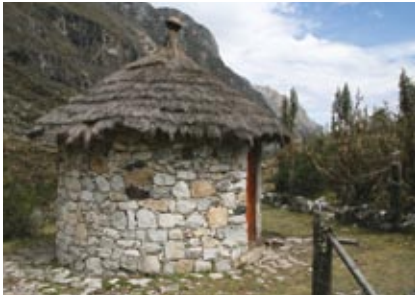
ABOVE HNP's toilets—an expensive (and ineffective) overkill.
