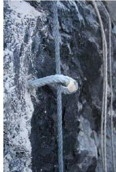
The eastern alp system with the tensioned cable running freely through the eyebolt
