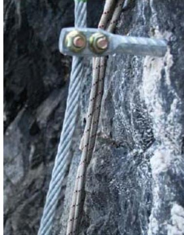
The eastern alps system with anchor clamps and a taut but untensioned cable
