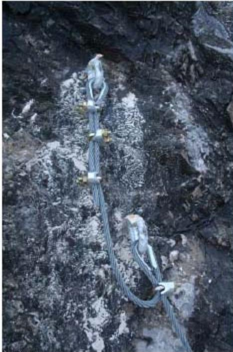
Fig 11 End anchoring for the French system
