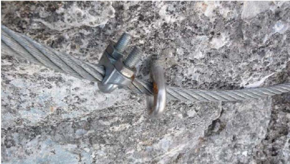
**Fig 17** Cable clamps on either side of an intermediate anchor limit wear.
