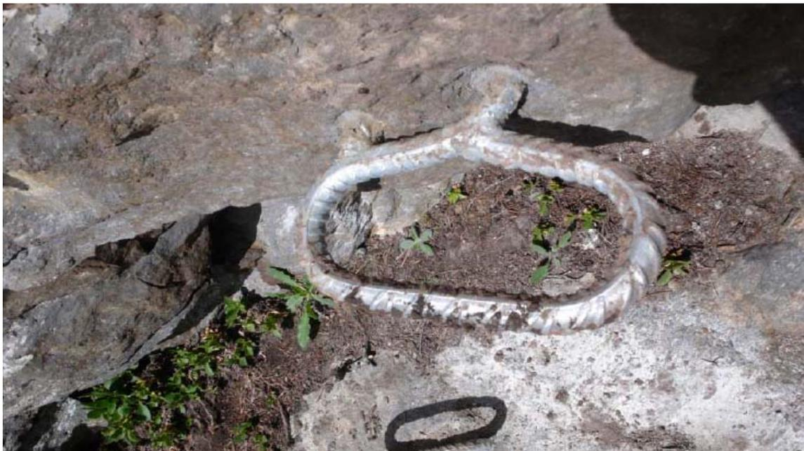
Fig 26 Foot pedals of galvanized, rebar steel—without burrs or sharp edges
